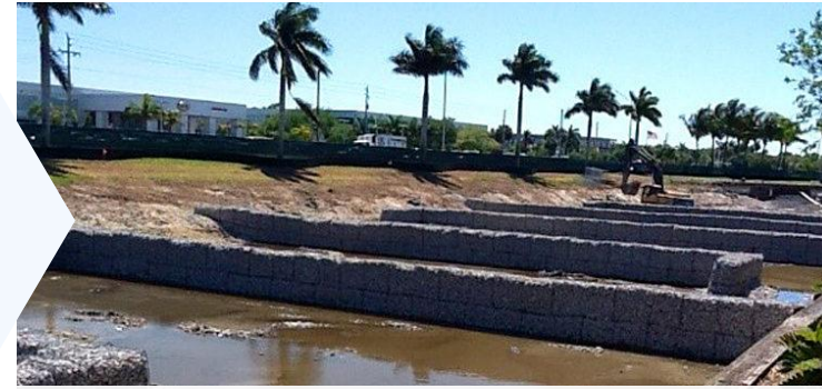
Pond 212 – Under Construction (2016)
