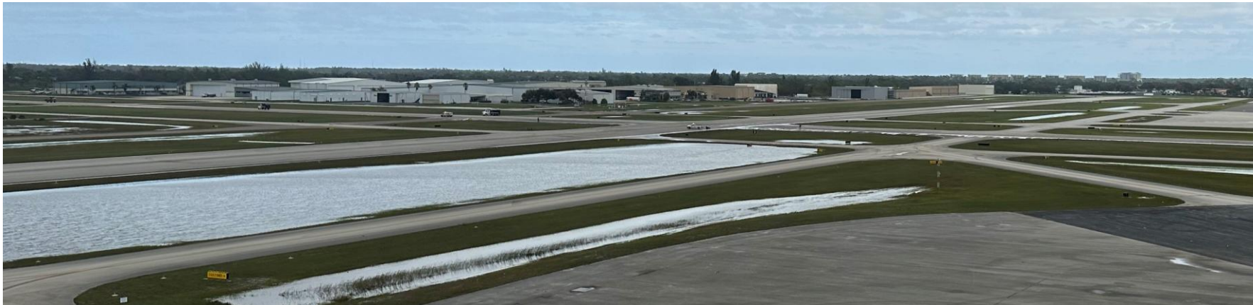
Runway 5-23 Drainage Improvements – Image taken after Hurricane Ian, September 29, 2022
